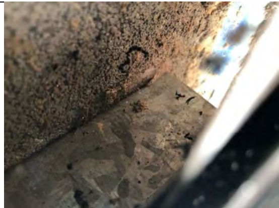
Photo 21: Sample number 122538 – behind panel view
