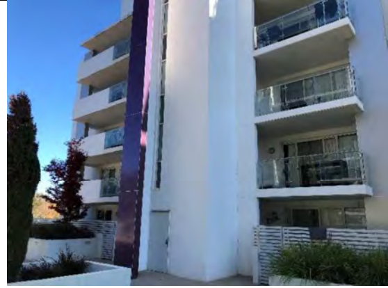
Photo 39: Sample number 122542 – façade view
