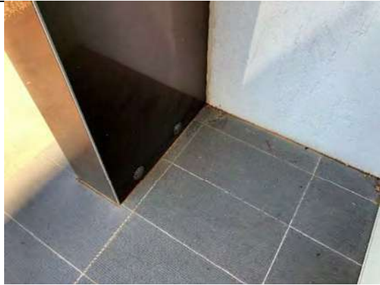
Photo 26: Sample number 122539 – sample location view
