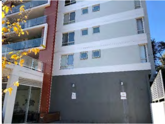
Photo 32: Sample number 122540 façade view
