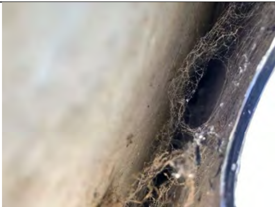
Photo 18: Sample Number 122537 – behind panel view
