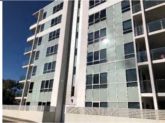
Photo 9: Façade from where sample 122534 was taken
