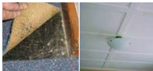
3. Internal areas wall and ceiling panels, carpet underlay, textured paints, insulation in domestic heaters
