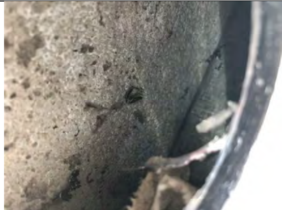
Photo 25: Sample number 122539 – behind panel view
