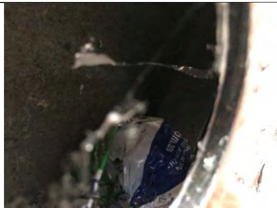
Photo 29: Sample number 122540 – behind panel view
