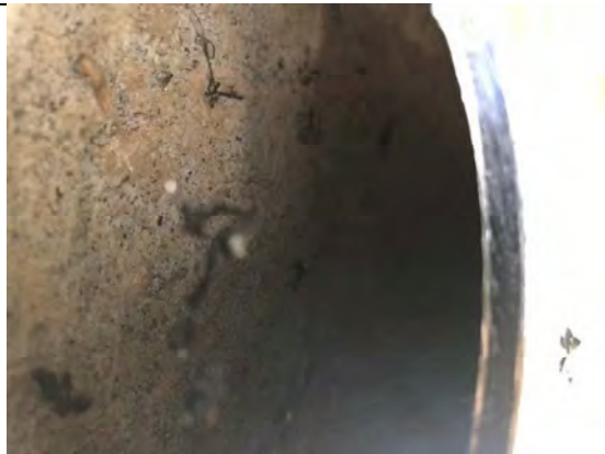
Photo 34: Sample number 122541 – behind panel view
