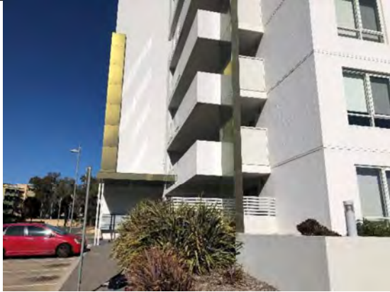
Photo 14: Façade view of where sample 122536 was taken.
