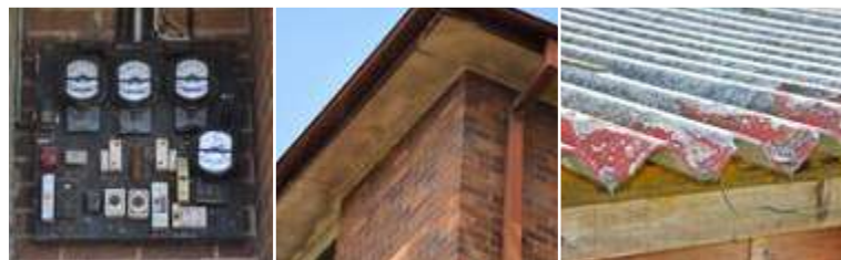
1. Exterior roof sheeting, gutters, downpipes, ridge capping, eaves, cladding, electrical switchboards
