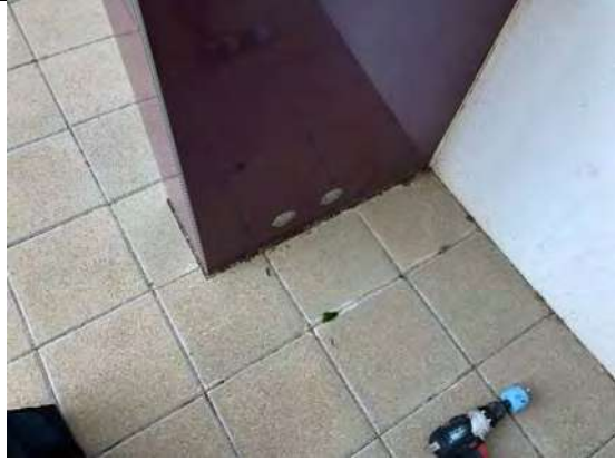
Photo 38: Sample number 122542 – location view
