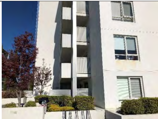
Photo 36: Sample number 122541 – façade view
