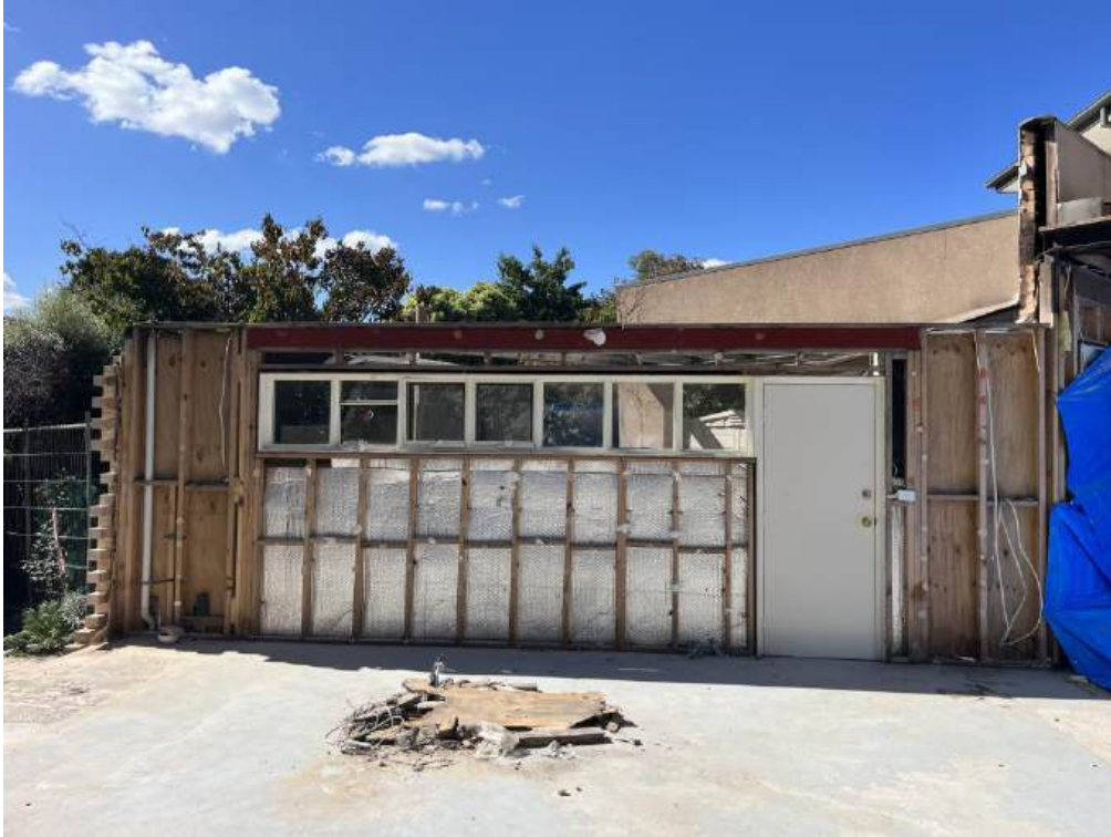
Image 3. View of the Brick Veneer Timber Stud Work to Removed and Replaced, Veneer to Remain in Place
