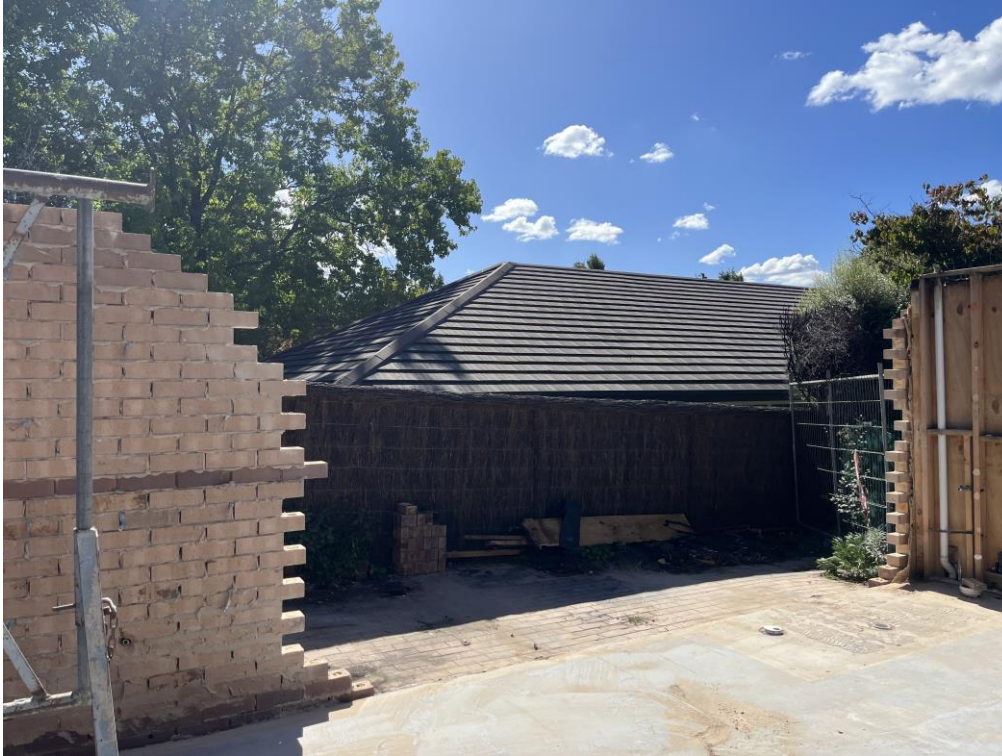
Image 2. View of the Existing Brickwork to Remain and New Brickwork to Integrate and Tooth Into
