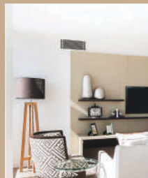
AIR CONDITIONING & MECHANICAL SERVICES
