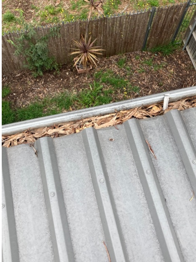
Photo 1.22 Before gutter clean
