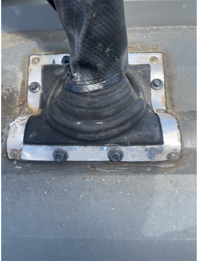
Photo 1.8 Additional fixings to existing boot type flashing
