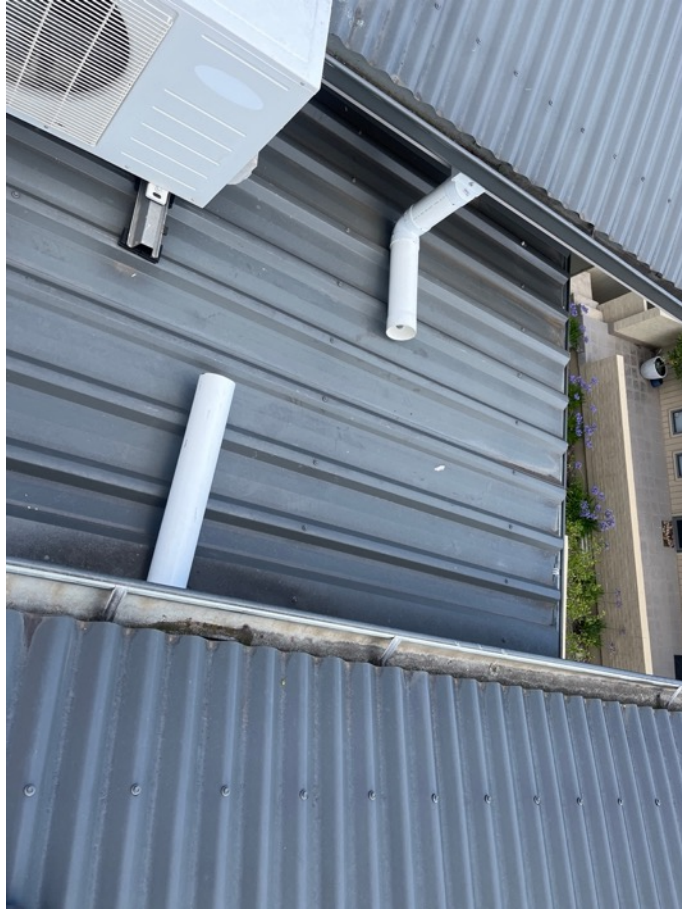
Photo 1.18 Installation of downpipe spreader
