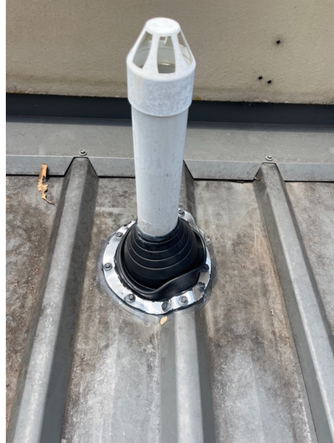
Photo 1.5 Completed boot type flashing
