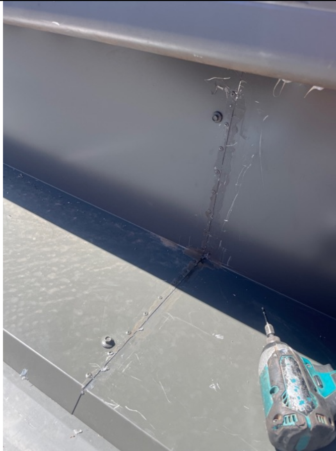
Photo 1.14 Strip and reseal join to flashing
