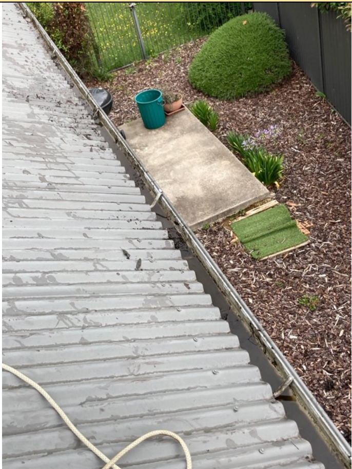
Photo 1.26 After gutter clean
