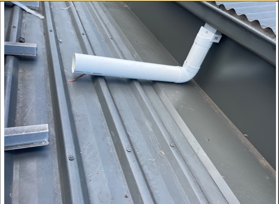
Photo 1.17 Installation of downpipe spreader
