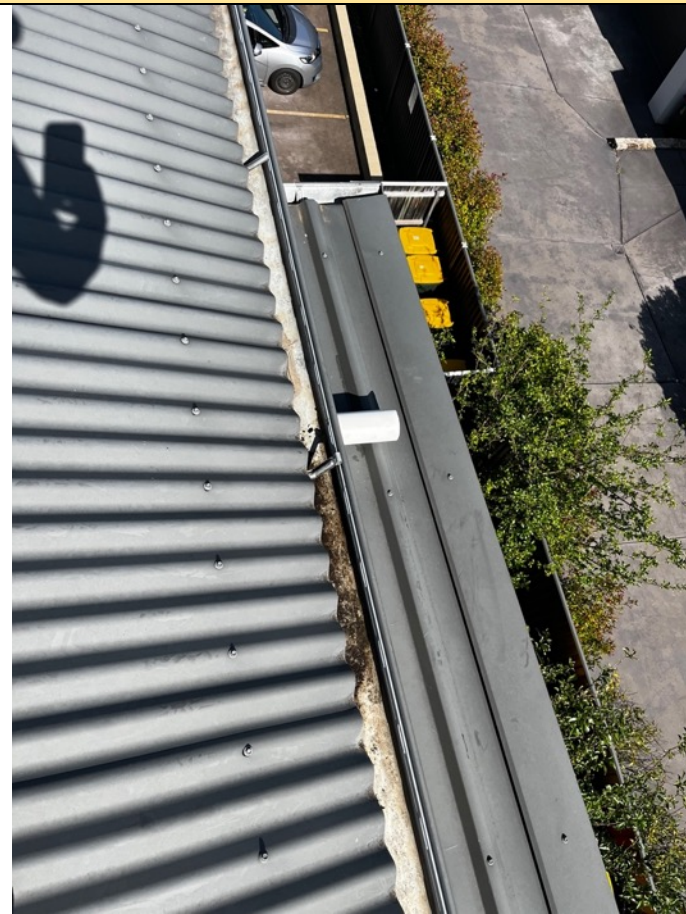
Photo 1.27 After gutter clean
