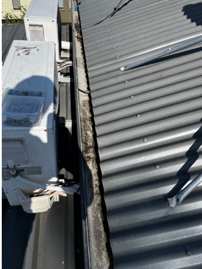
Photo 1.24 After gutter clean
