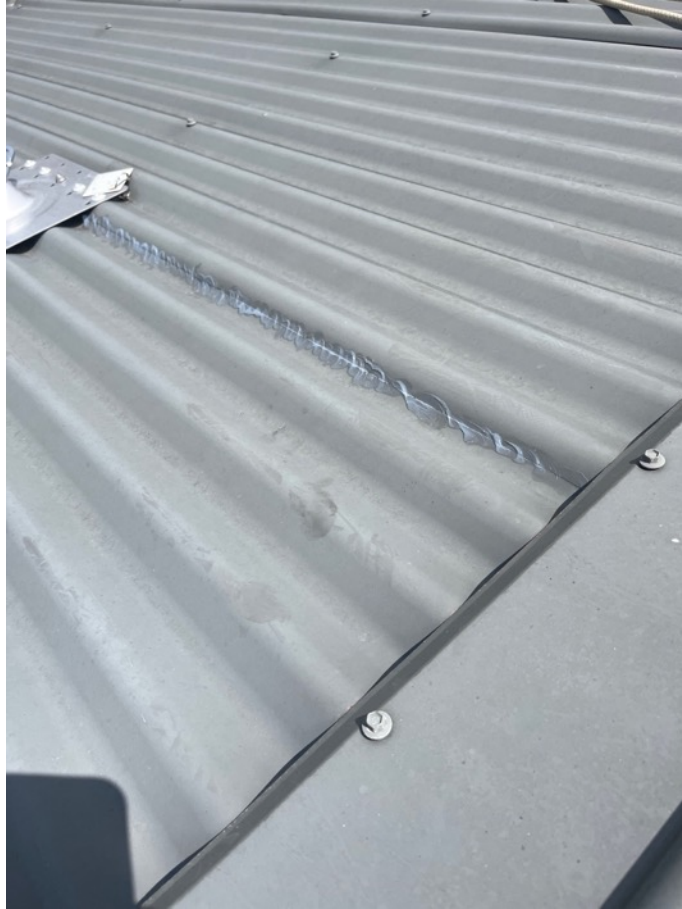
Photo 1.20 Seal lap to the head of the roof
