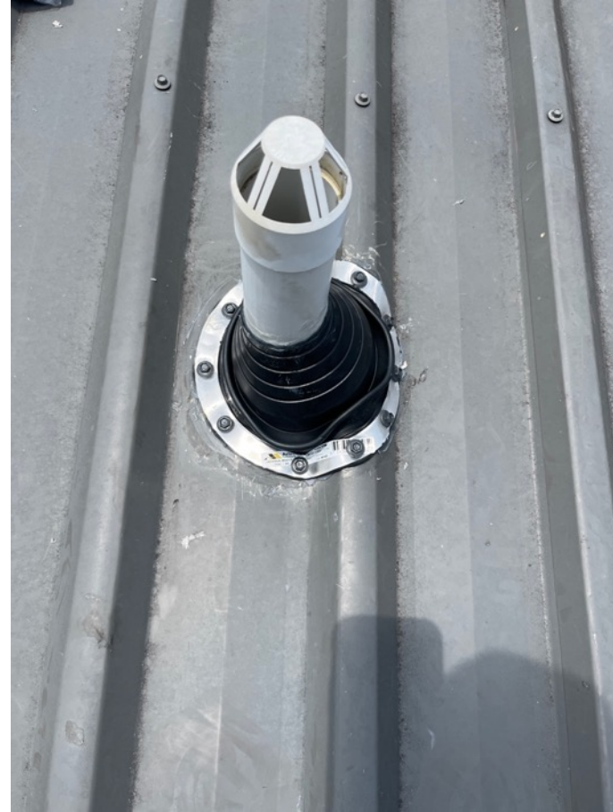
Photo 1.7 Completed boot type flashing
