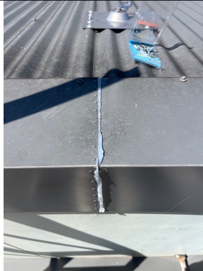
Photo 1.15 Strip and reseal join to capping
