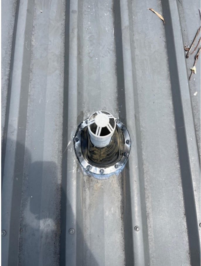
Photo 1.6 Completed boot type flashing
