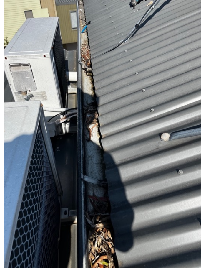
Photo 1.21 Before gutter clean
