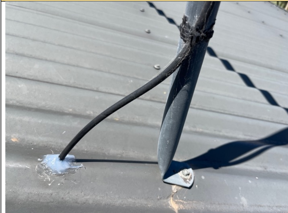
Photo 1.16 Strip and reseal cable penetration
