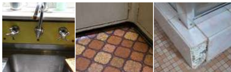
2. Wet areas - bathroom, laundry and kitchen wall and ceiling panels, vinyl floor tiles, backing for wall tiles and splashbacks, hot water pipe insulation
