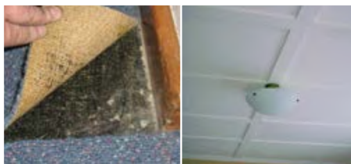
3. Internal areas wall and ceiling panels, carpet underlay, textured paints, insulation in domestic heaters
