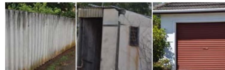
4. Backyard fences, sheds, garages, carports, dog kennels, buried or dumped waste, letterboxes, swimming pools
