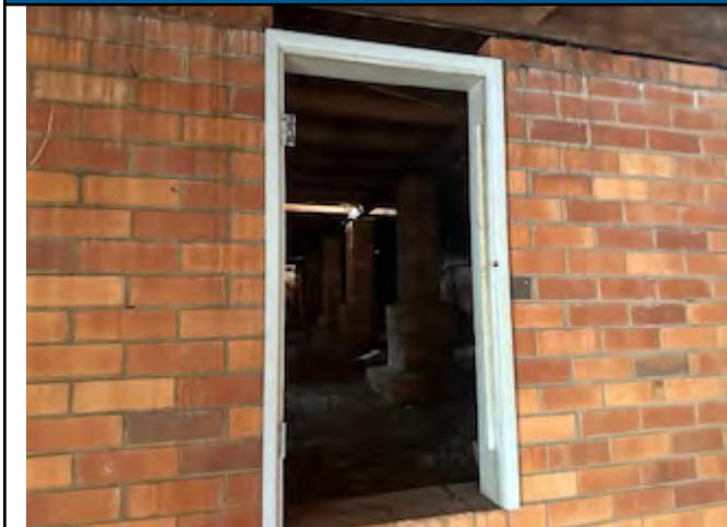
REMOVAL WORK AREA
