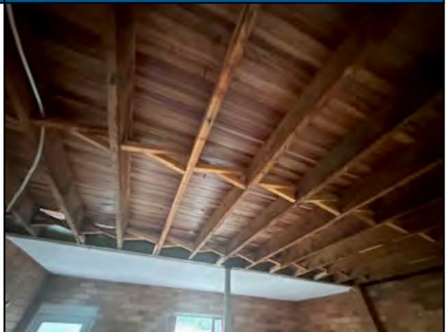
REMOVAL WORK AREA
