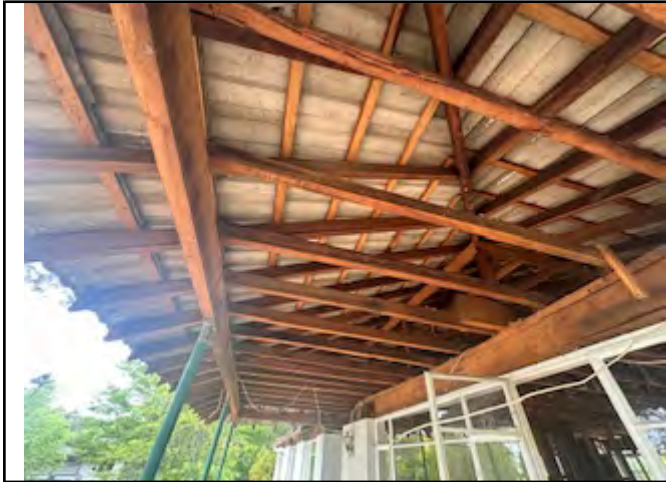
REMOVAL WORK AREA
