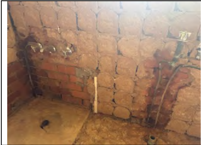
REMOVAL WORK AREA
