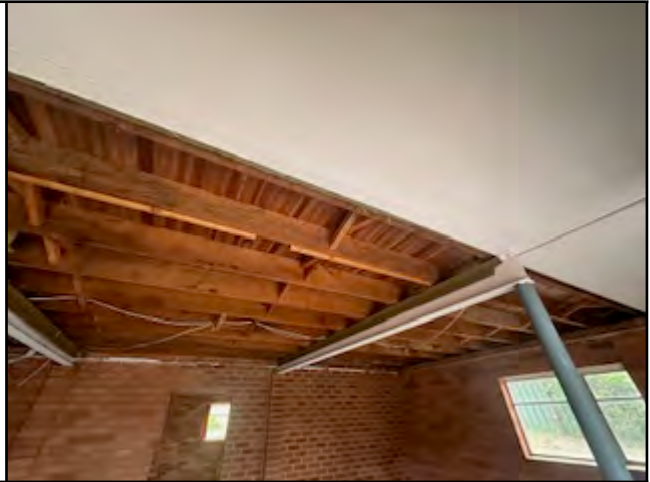
REMOVAL WORK AREA
