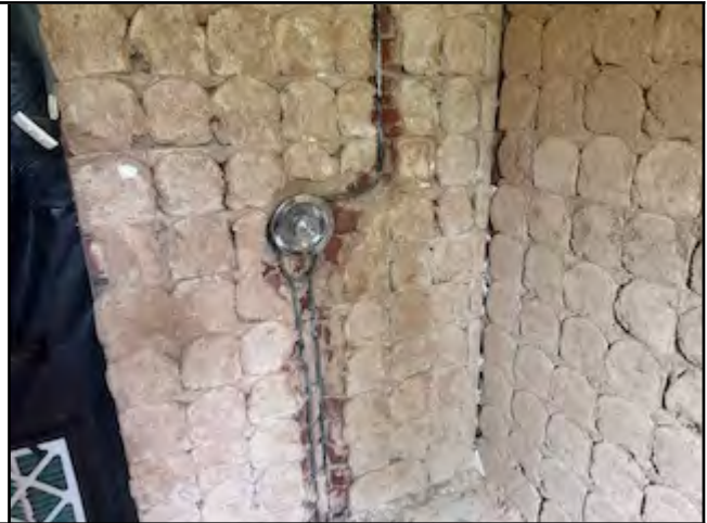
REMOVAL WORK AREA
