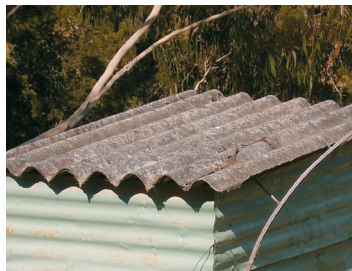
Corrugated asbestos roofing
